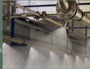
WATER SPRAYING SYSTEM for HOLD
