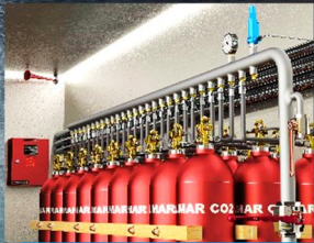
CO 2 FIRE EXTINGUISHER
