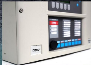
FIRE DETECTION SYSTEM
