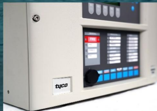
FIRE DETECTION SYSTEM
