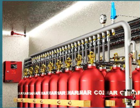
CO 2 FIRE EXTINGUISHER
